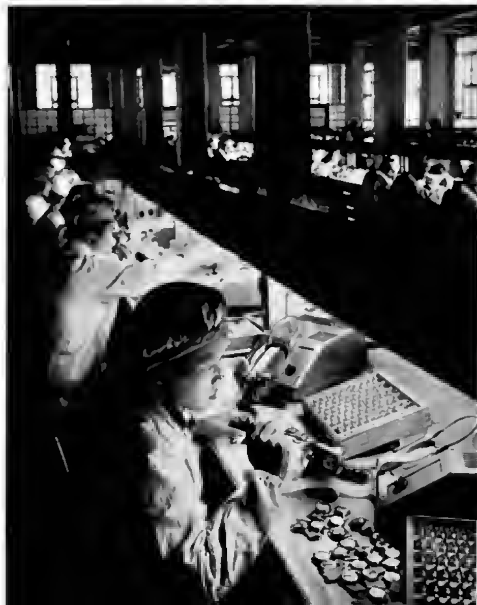
Workers at the Shanghai Wrist Watch Plant check the performance of watches made with domestically produced jewels and hairsprings.
